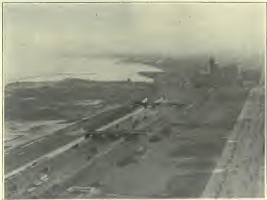
FIG. 330. FREIGHT YARDS. Jackson Street Yard of the Illinois Central Railroad.
